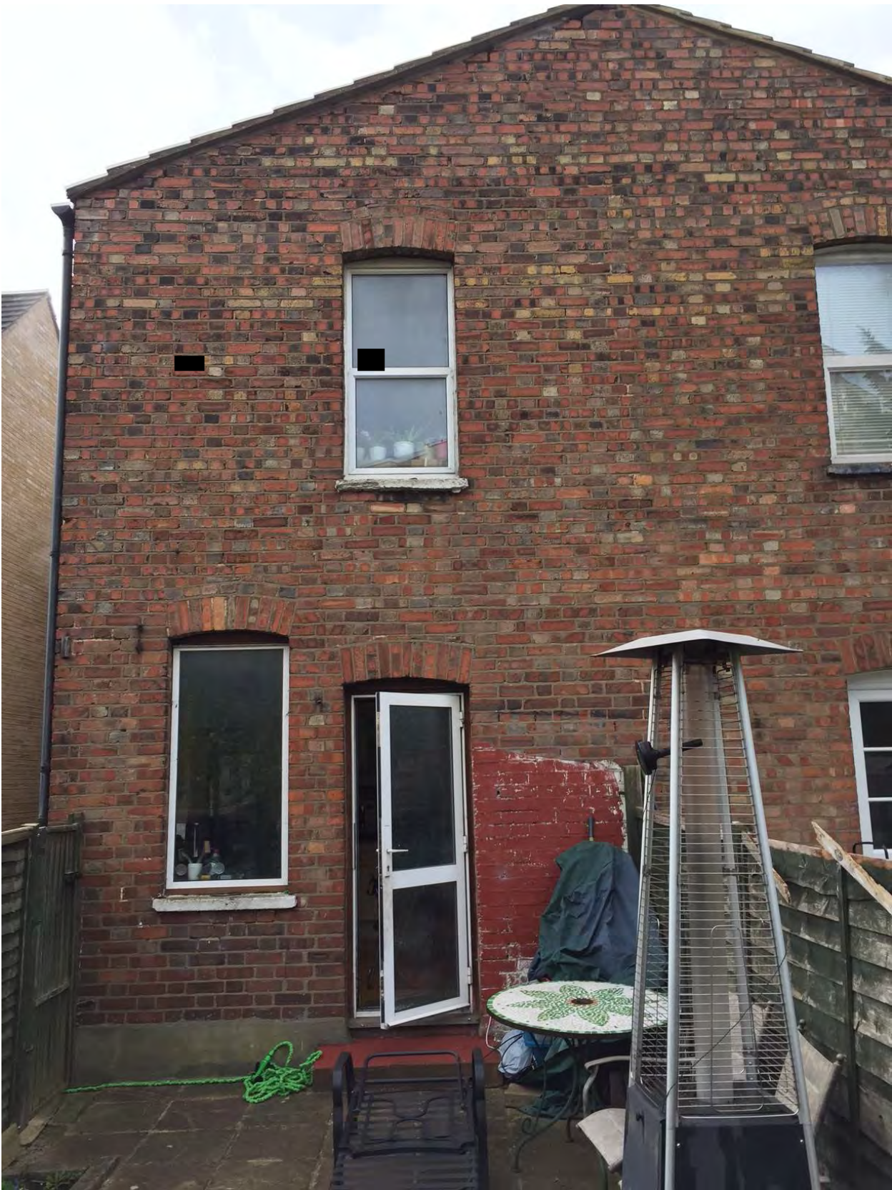
Existing rear elevation of No.2 Vaughan Road.
