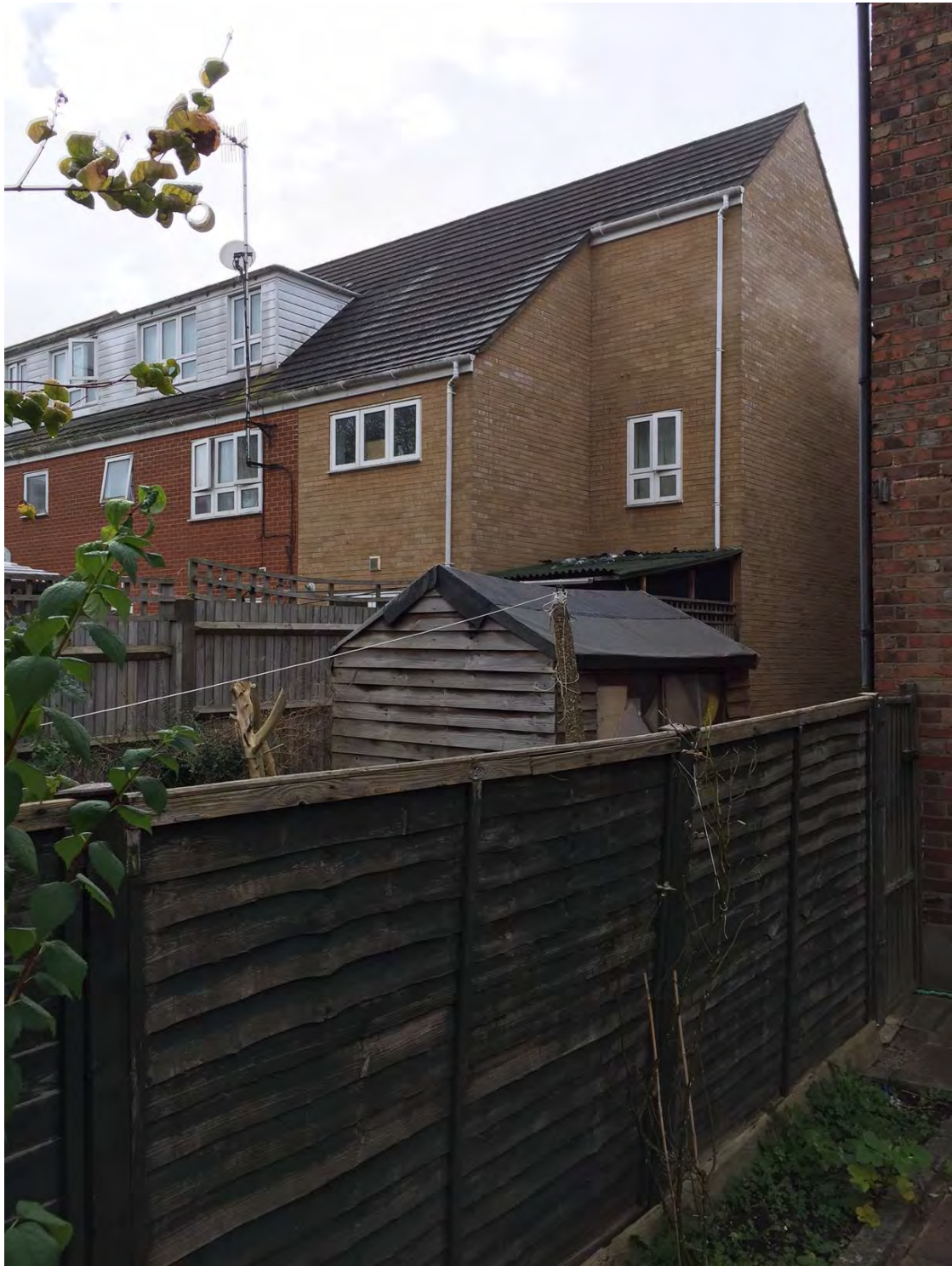
Rear elevation of the neighbouring dwellinghouse, No.2A Vaughan Road
